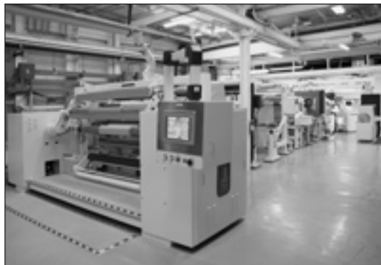
Extrusion Coating Lab - Fulton, NY
